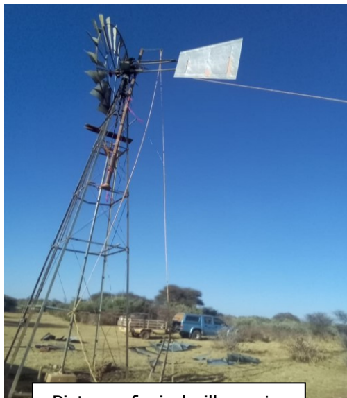
Picture of windmill repairs
